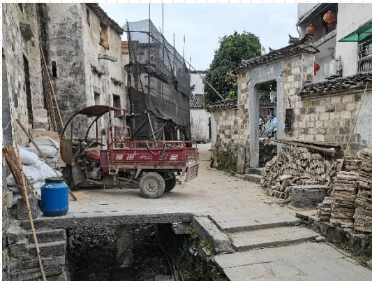
Construction of Houses
